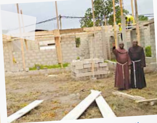
Br. Severin and Br. Nicodemus at the school site, in front of the classrooms under construction.
